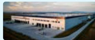
ACCOLADE FUNDS PARK KOŠICE AIRPORT
